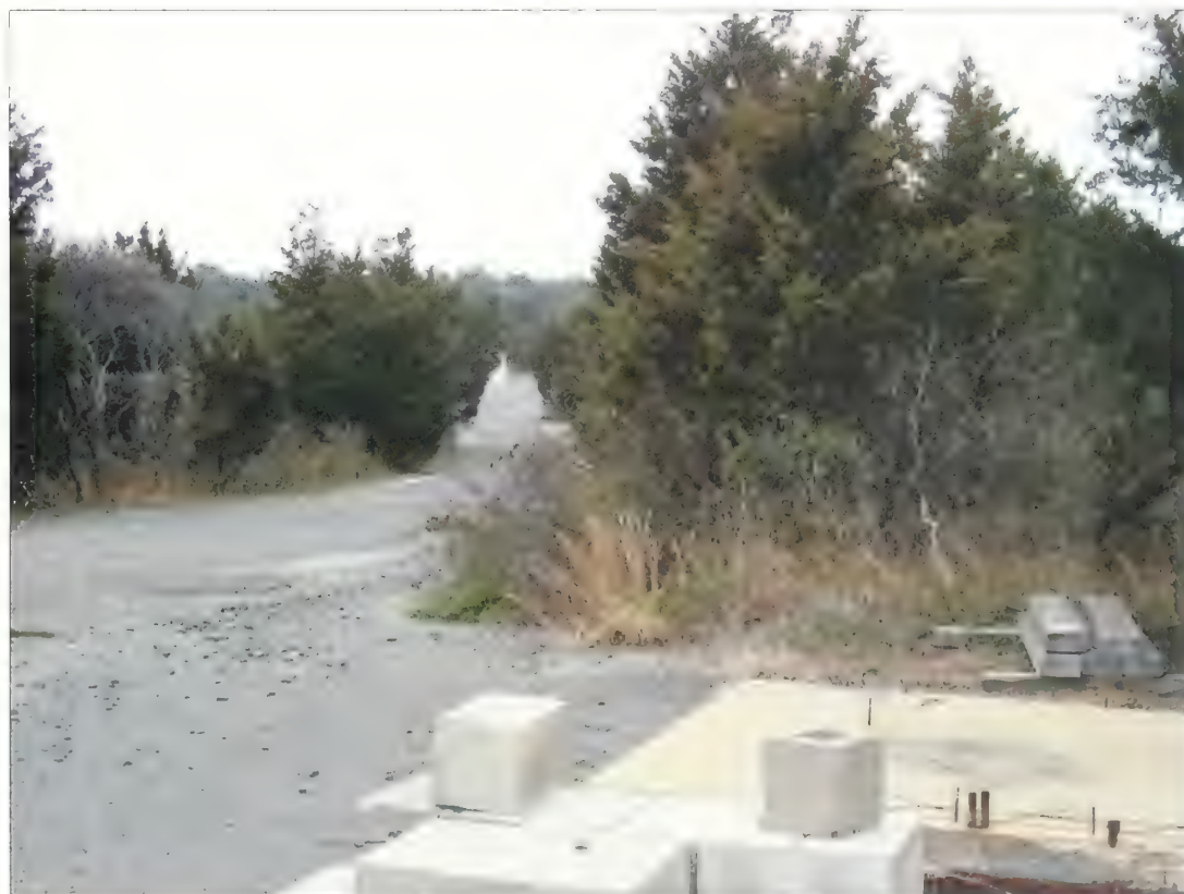
Figure 5.125. View looking northwest toward the Ready Barracks, NIKE launch site. The sentry hut near the missile magazines should be reconstructed as part of plans to prepare the site for visitor access and interpretation. The concrete foundation for the hut is visible in the right foreground (Olmsted Center, April 2008).
